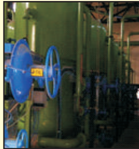
SOFTENING PLANT Capacity : 3 x 120 m 3 /hr 10 x 120 m 3 /hr 12 x 120 m 3 /hr
