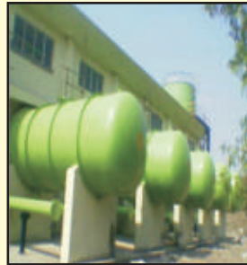
FILTRATION PLANT Capacity : 3 x 120 m 3 /hr 10 x 120 m 3 /hr 12 x 120 m 3 /hr
