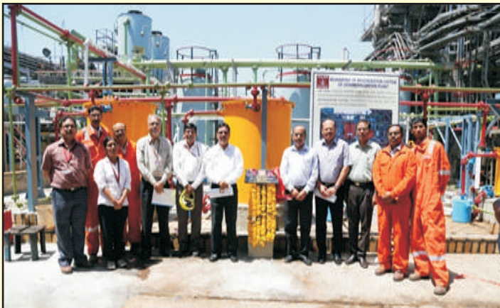
Revamping of DM Plant regeneration Systems at ONGC Hazira, Gujarat
